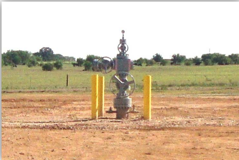
Wellhead - Desalination Concentrate Disposal Well (San Antonio Water System)
